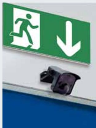
Radars detector in escape direction as standard
